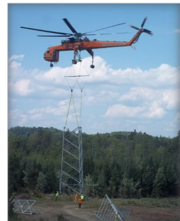
Figure 6: Sky Crane Lifting Communication Tower
